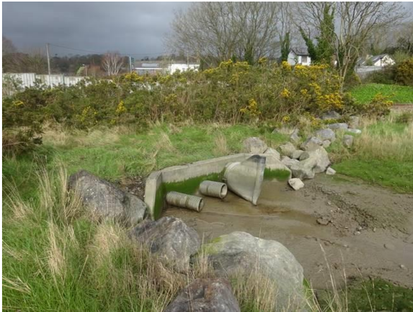
Figure 2-4 – Existing Outfall east of Glounthaune Train Station at Johnstown Park
