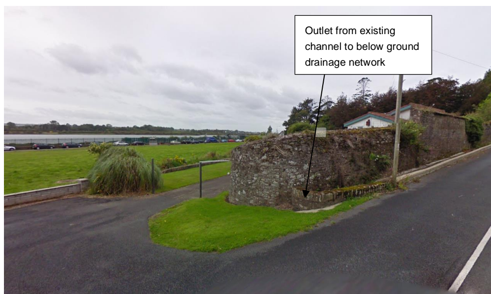
Figure 2-2 – Existing Channel on the Terrace/ Johnstown Close
