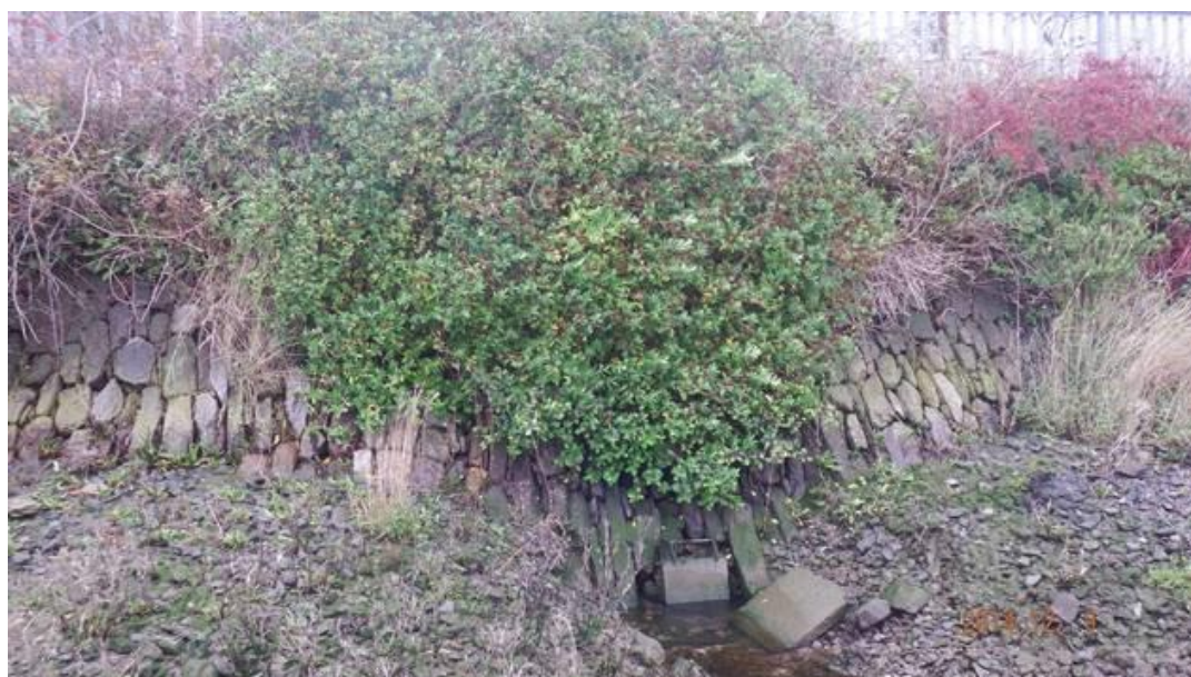
Figure 2-3 – Existing Outfall at Glounthaune Train Station
